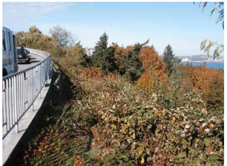
Transition planting needed at crest of slope
