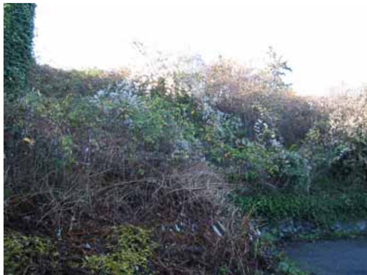
Overgrown vegetation from toe of slope
