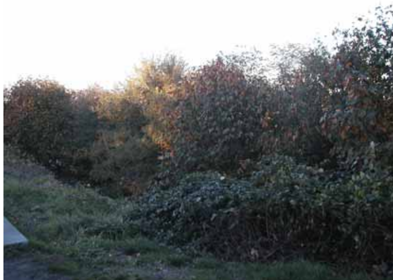
Invasive vegetation dominates crest of slope
