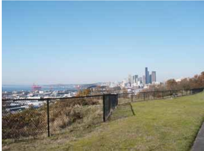
Transition area at crest of slope, looking North.
