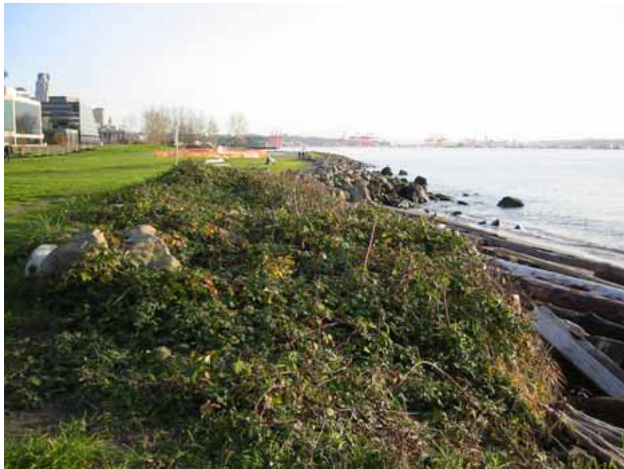
Invasive weeds growing along crest of slope at shoreline
